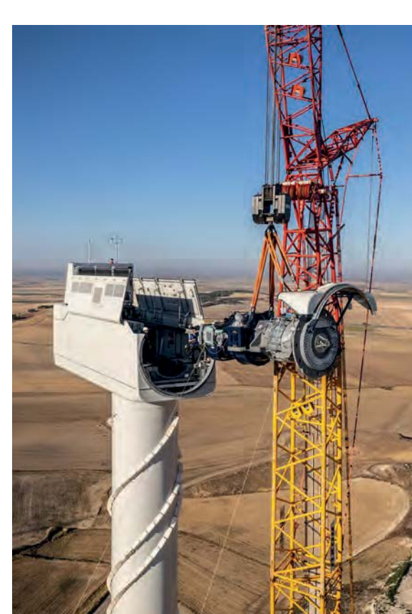
The drive rod is installed
