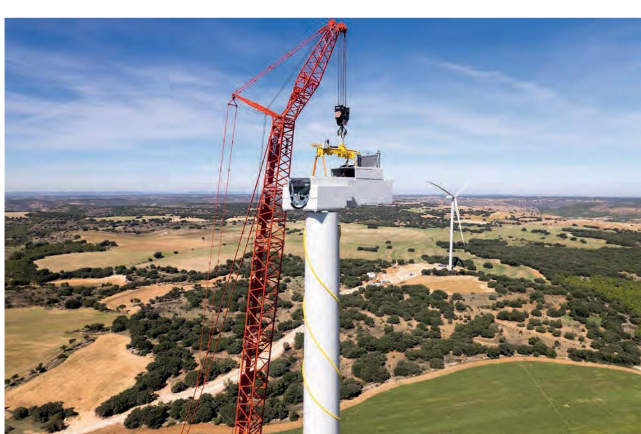
Once the tower has been erected, the gondola is placed on top
