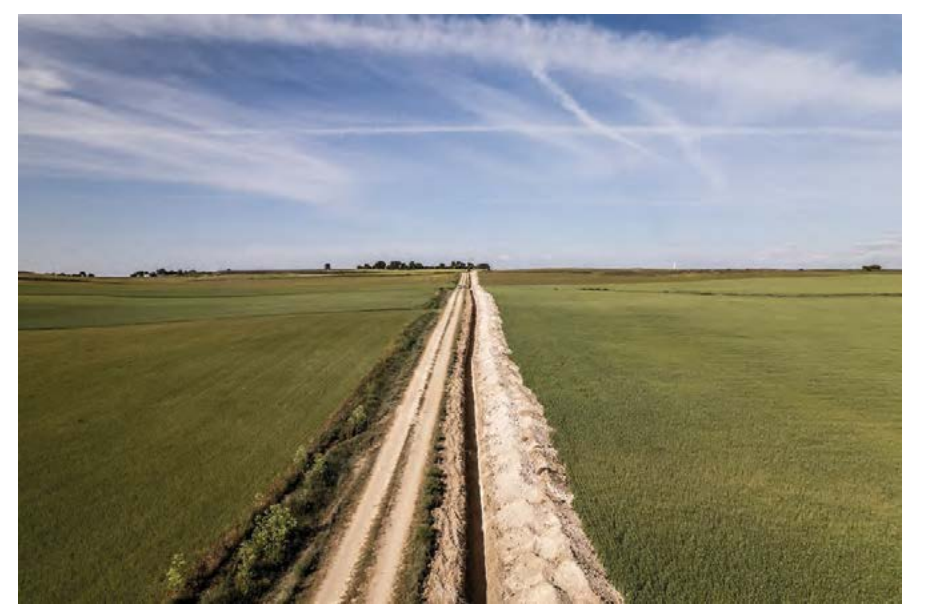
Trench for collector line
