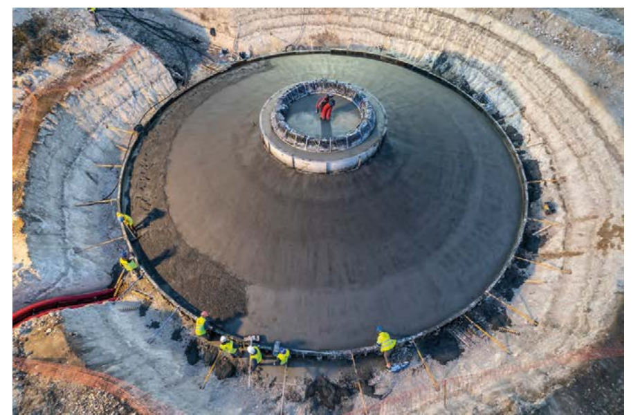
Concreting of foundations (500-600 m 3 per wind turbine)
