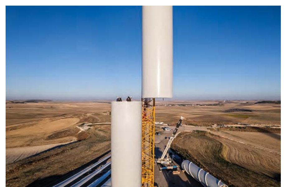
Fitters take delivery of a new segment and adjust it
