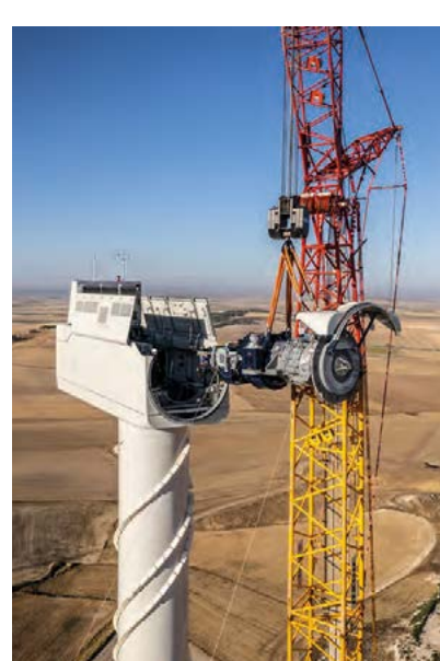
The drive rod is installed
