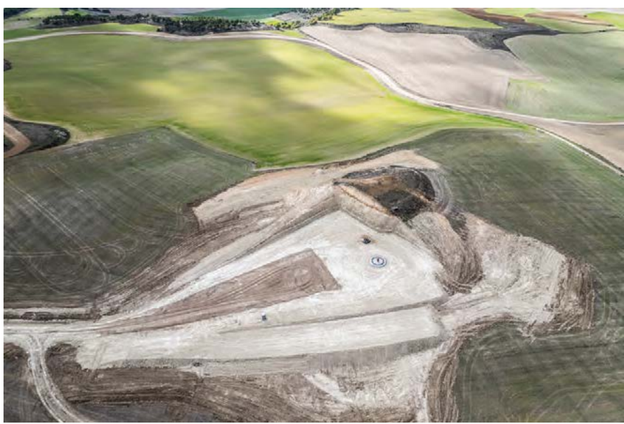
Ground movement on platforms
