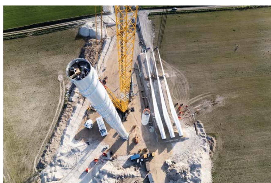
The tower segments are installed one after the other
