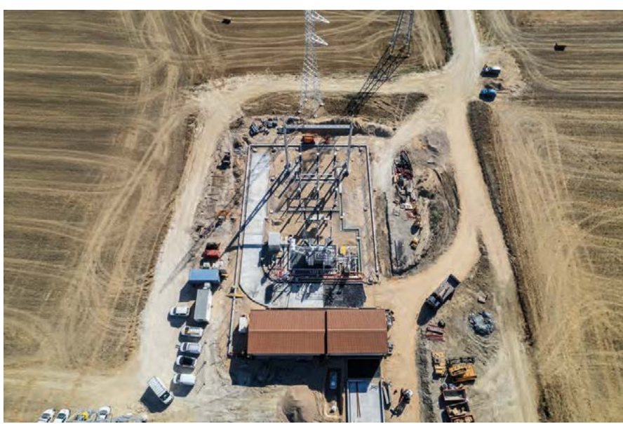
Construction of the transformer substation
